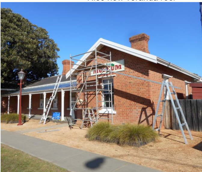
Nice new veranda roof
