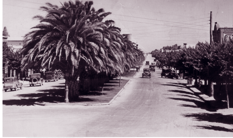
■ Looking South along High Street (Circa 1930)
