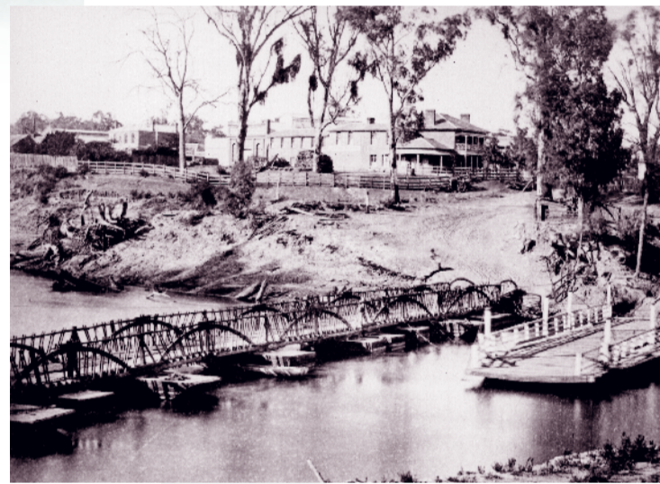
■ Hopwood's Punt and Bridge Hotel (Circa 1865)
